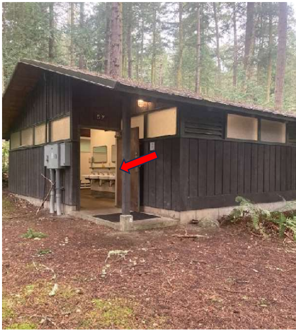
Bathroom for outdoor classroom
